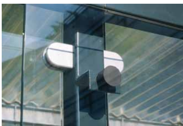
Detail glasinklemming
