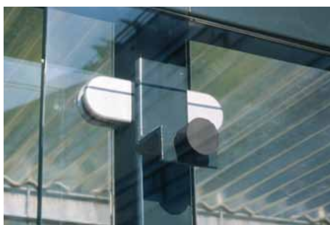
Detail glasinklemming
